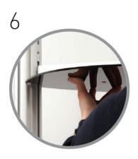
Ensuring the black acrylic is lowermost, slide and raise second assembly into the same post channels as the previous enclosure until the expanding clamps come into contact with the bottom of the pre-installed locator bars of the upper posts. Tighten grub screws in ends of profile to secure in position.
