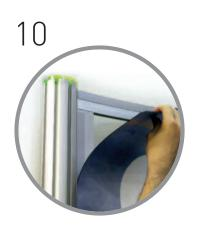
Affix graphic panels to the graphic fixing strips, starting from the top and side, working across the completed system.
